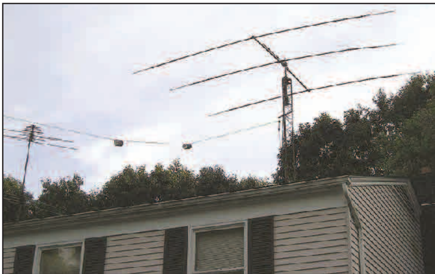
Figure 1 — W8NX Special antenna mounted at 47 feet on tower used to hold triband Yagi. This is an efficient antenna system that covers 160/80/40/30/17/12 meters with the dipole and 20/15/10 meters with the triband Yagi.
